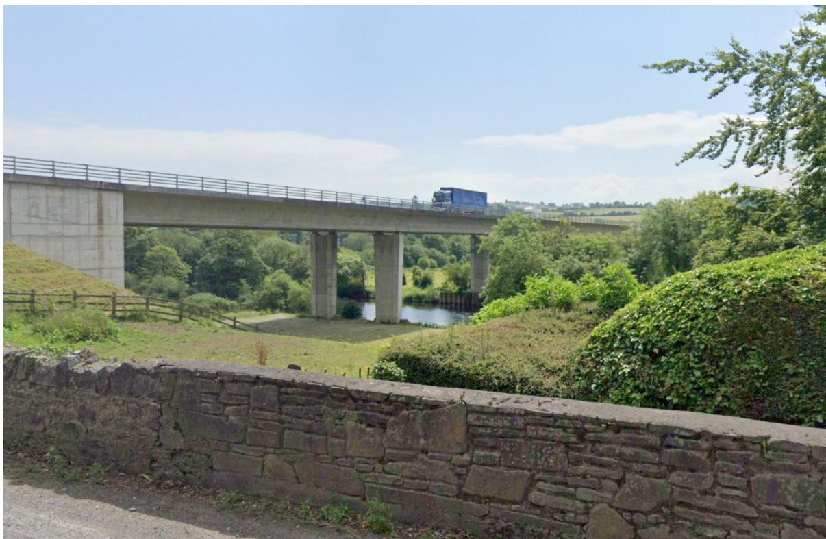
Figure 2-2; Google Streetview of M8 Bridge
