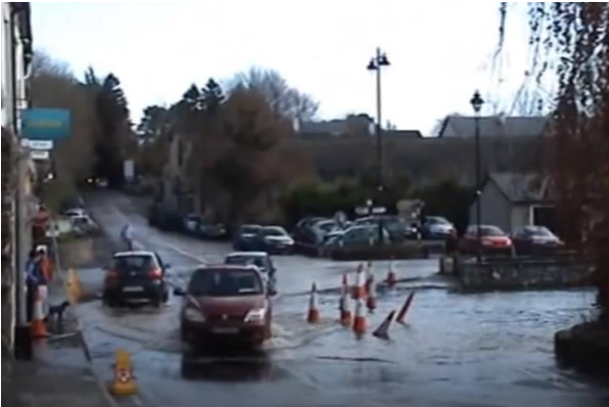
Figure 6-5: November 2009 Flooding - Road Junction
