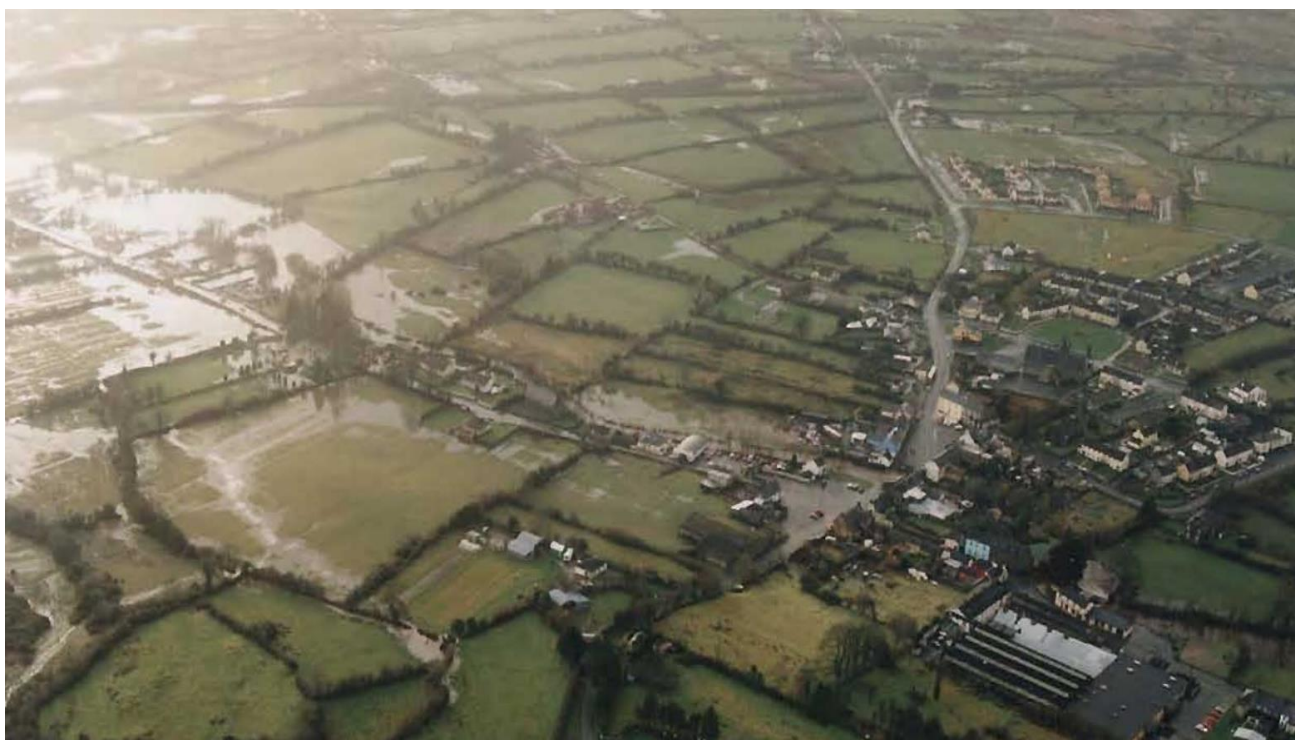
Figure 6-8: 1995 Flood Event - Sixmilebridge Village
