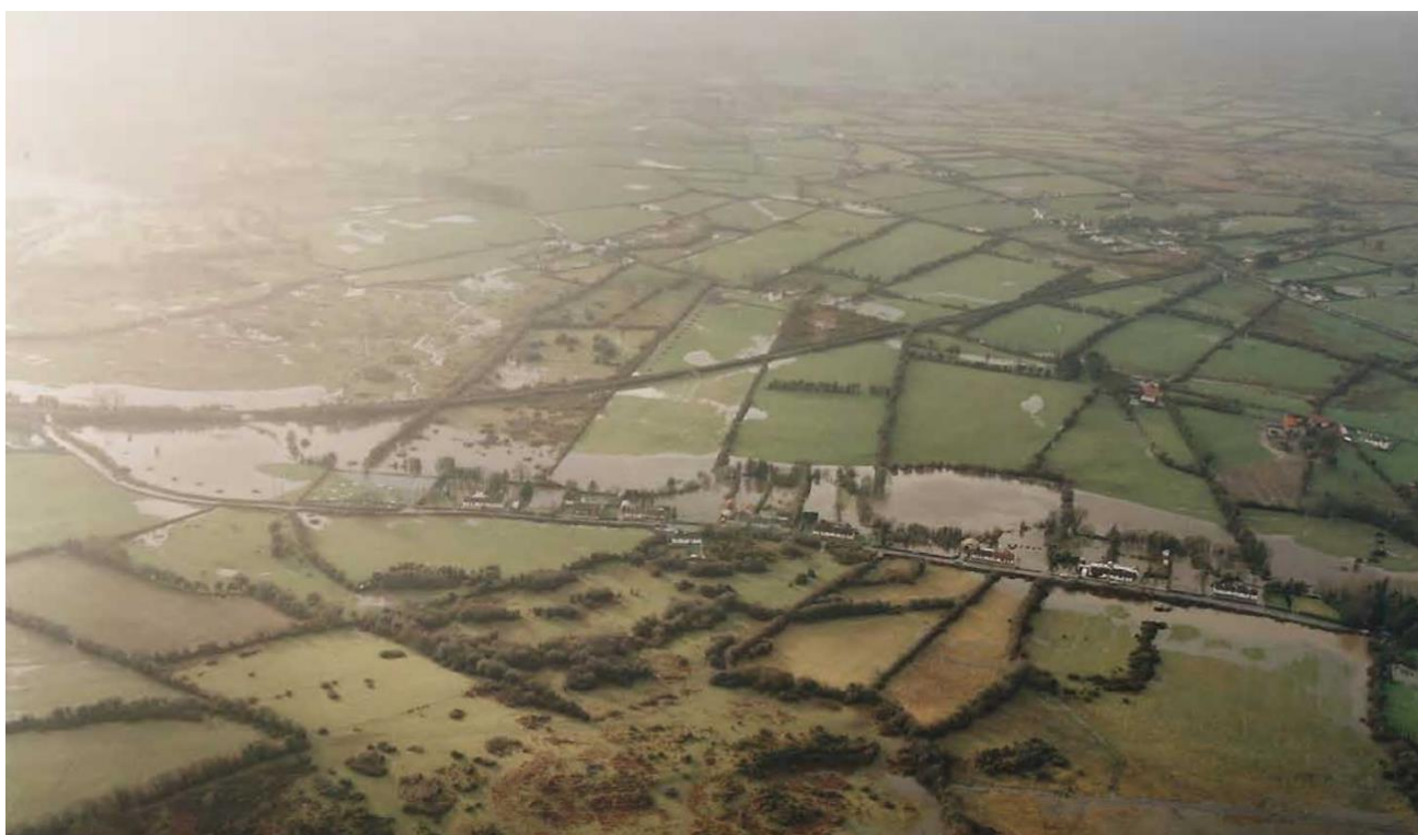
Figure 6-9: 1995 Flood Event - Downstream (Railway Crossing)
