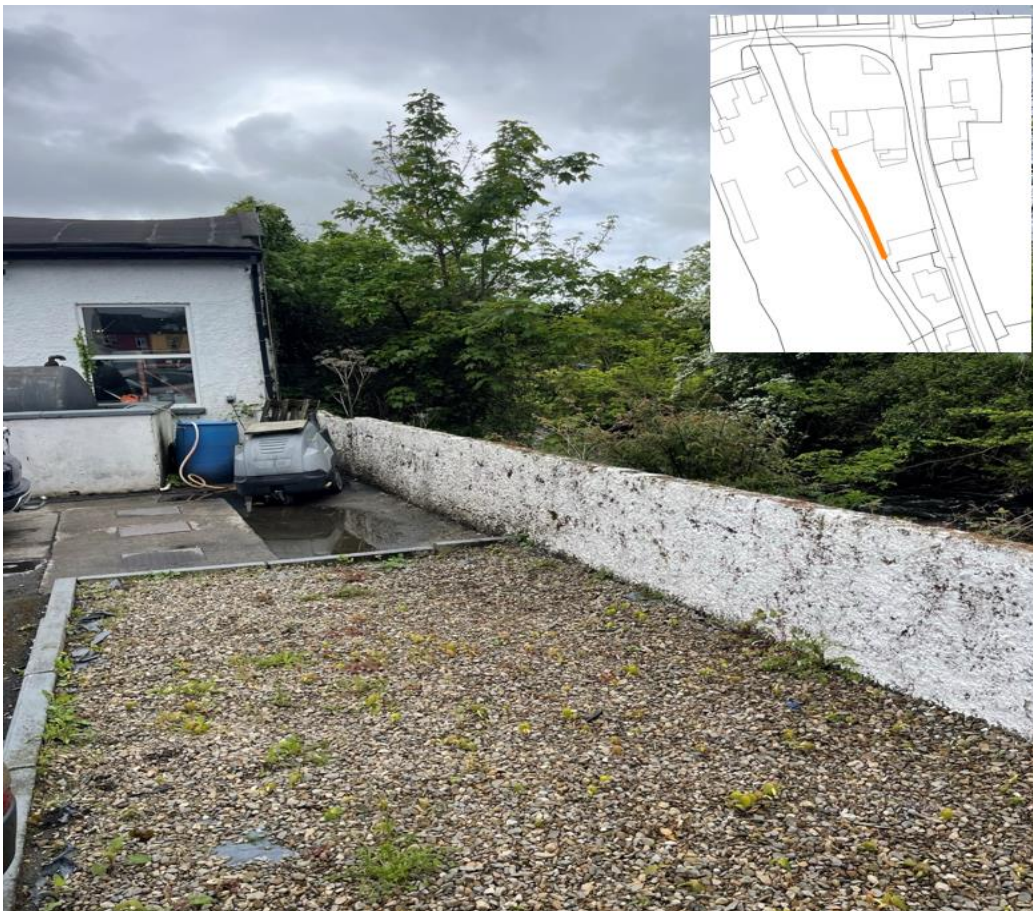
Figure 8-3: Wall removal - Left bank wall adjacent to the car park
