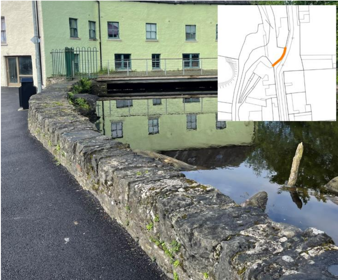
Figure 8-1: Wall removal - Mill pond roadside wall
