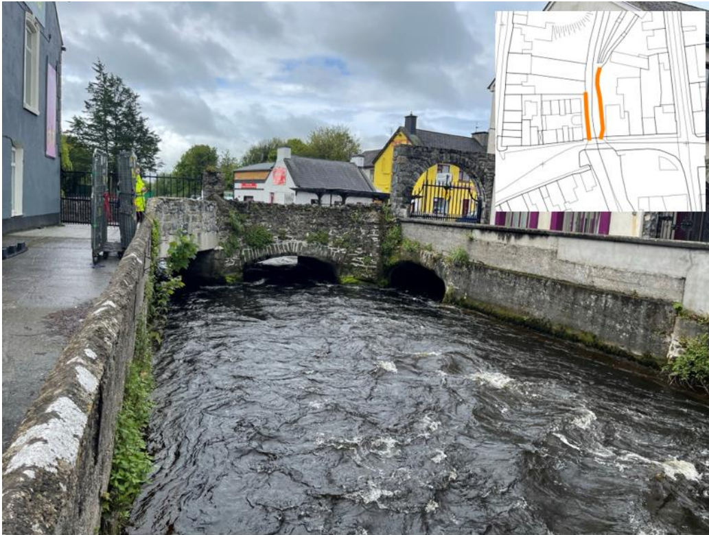
Figure 8-2: Wall removal - channel bank walls upstream of the road bridge
